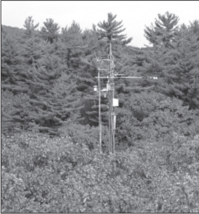
View of EMS tower.
