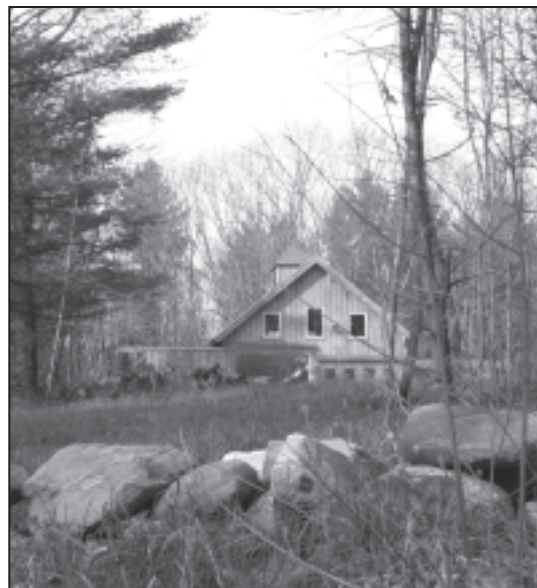
New maintenance garage on Prospect Hill.
