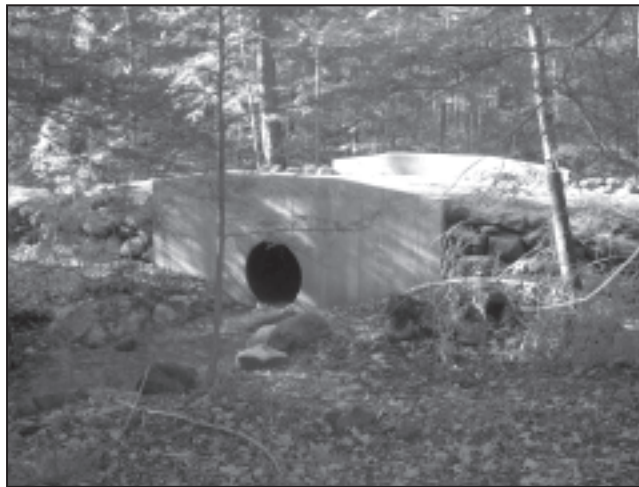
Culvert built in the fall of 2006 on Bigelow Brook.
